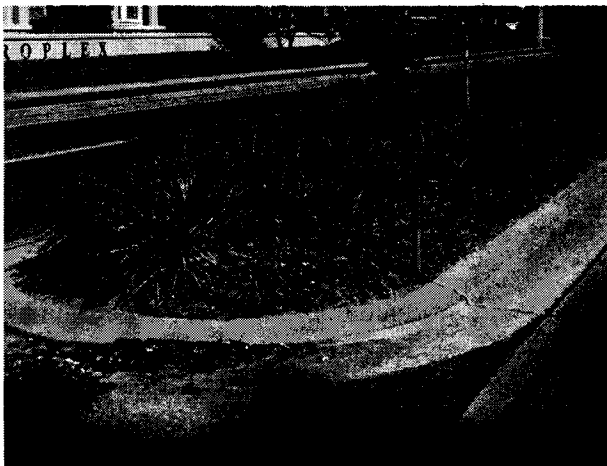
Figure 32 Median graded too high on 43 rd Street
