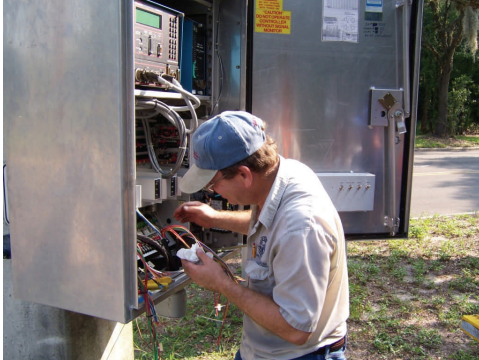
Technician working on traffic signal
