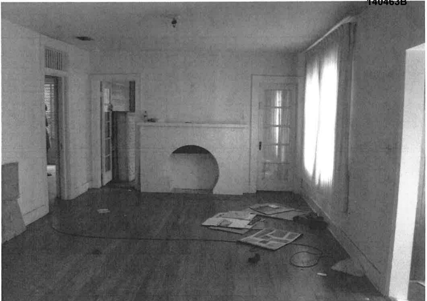
TYPICAL INTERIORS - HOUSE #2 (RANCH) - UNIQUE FIREPLACE TO BE SAVED.
