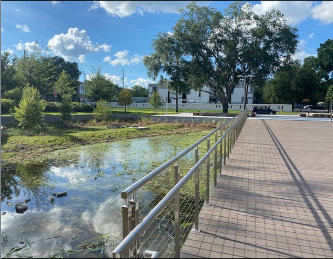
Pedestrian bridge over stormwater retention pond
