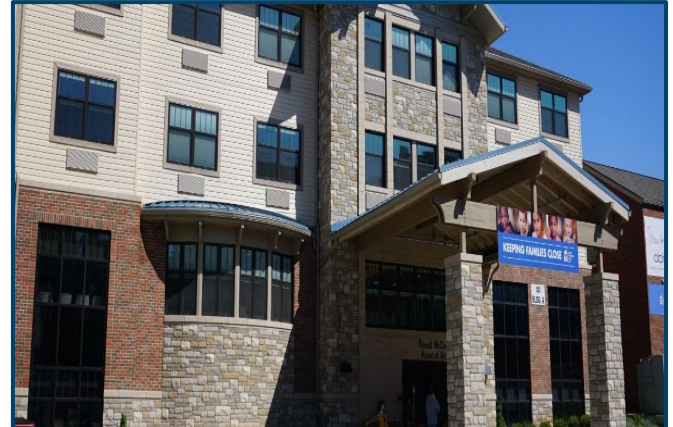
RONALD MCDONALD HOUSE OF AKRON NON-PROFIT PROJECT EXPERIENCE
