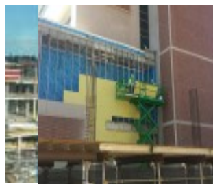
Panels are removed to allow the new hospitals to connect to the UF Health Shands Cancer Hospital.
