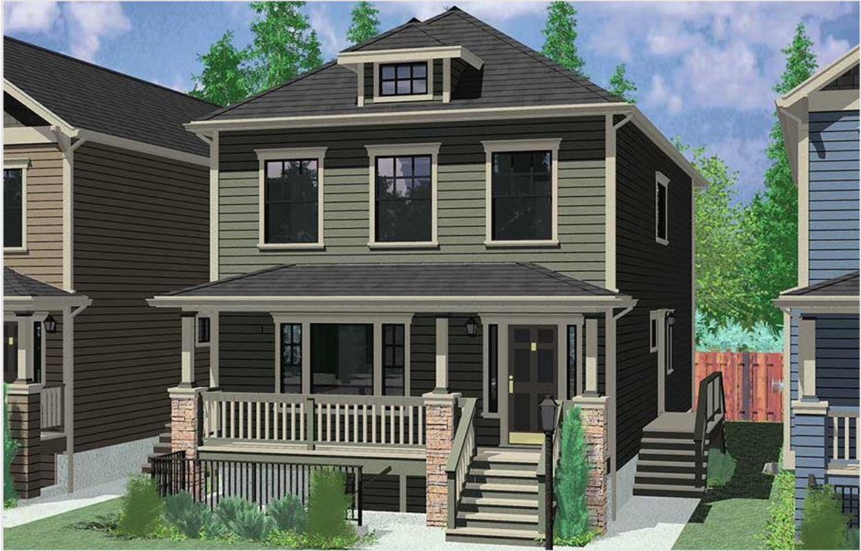
Example of a “stacked duplex” house plan from a Portland, Oregon Building Design Firm
