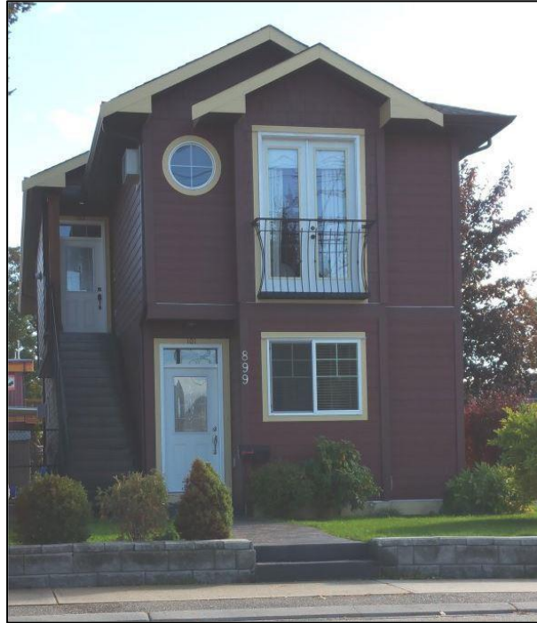
Example of a constructed vertical two-family dwelling
