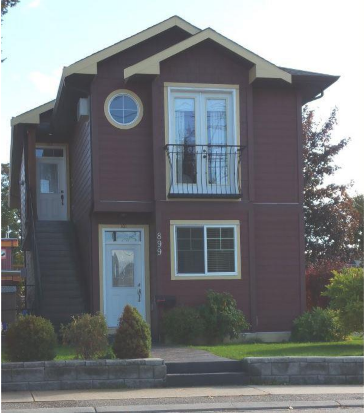
Example of a constructed “stacked duplex”
