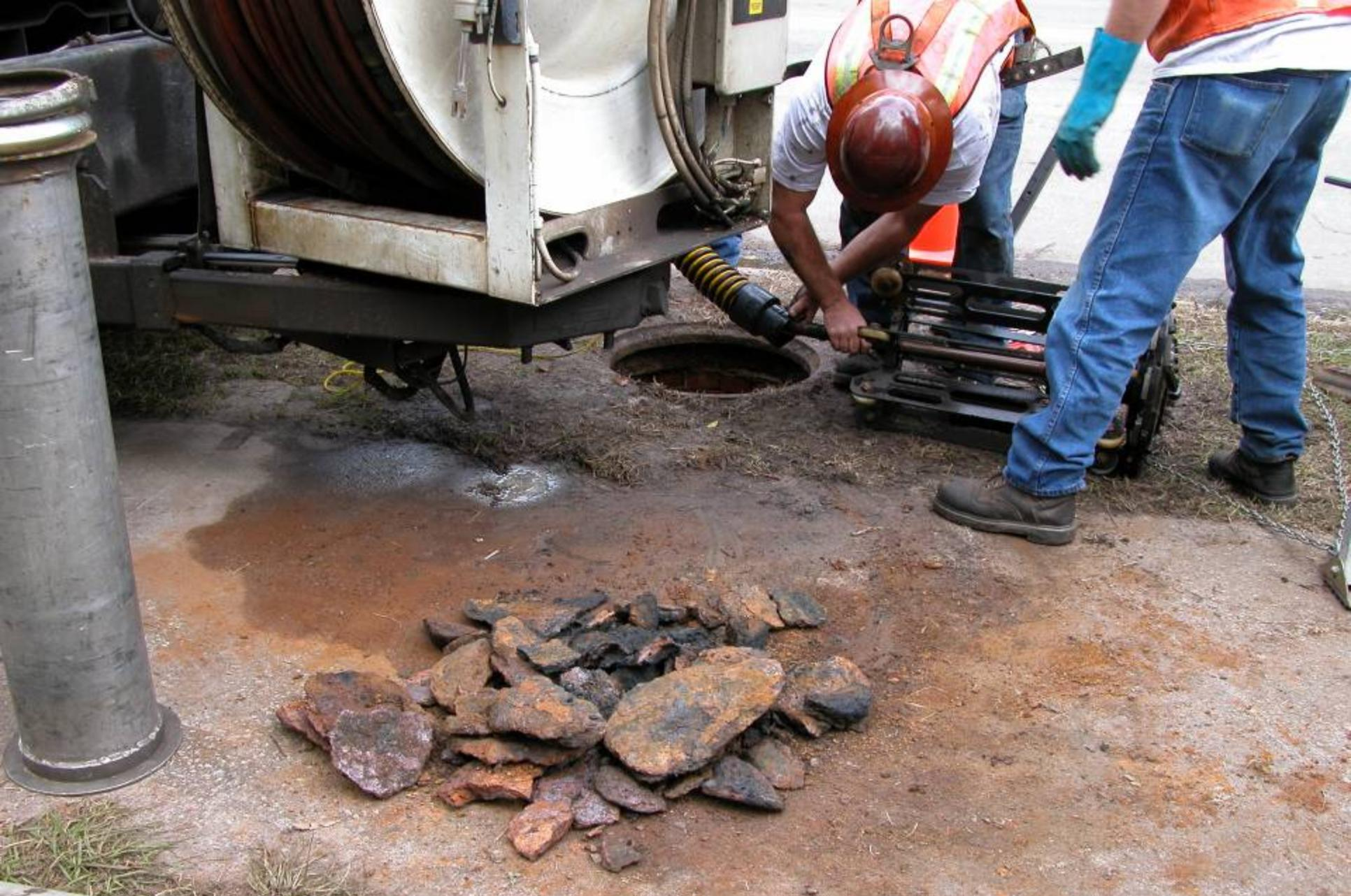
**Tuberculation Removed with Hydraulic Chain Cutter**
