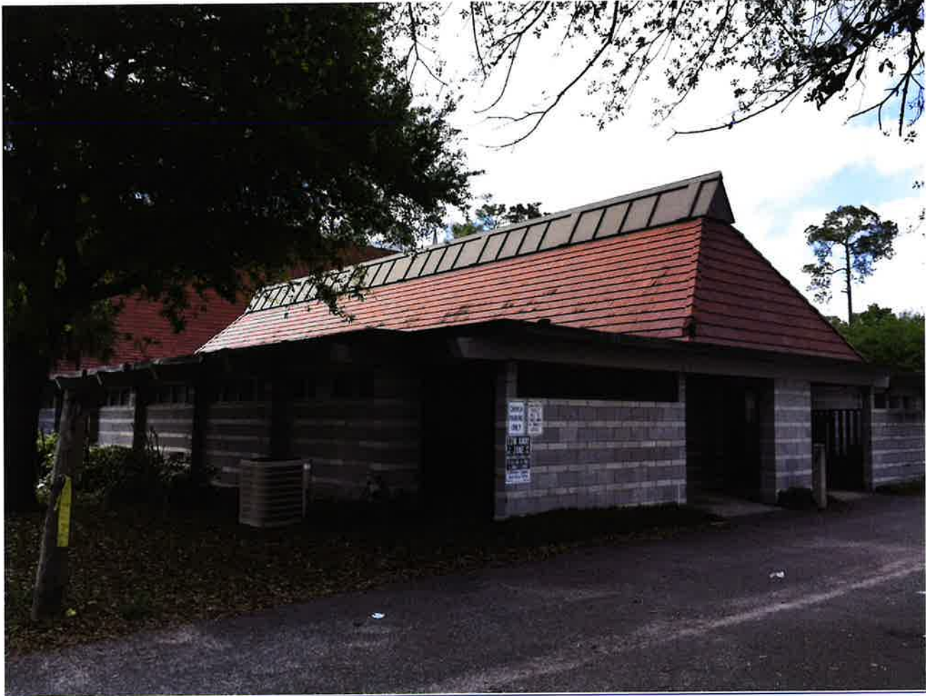
Figure 8. Lutheran Campus Center, Ludovici tile roof. Image Sujin Kim, photographed September 7, 2016.
