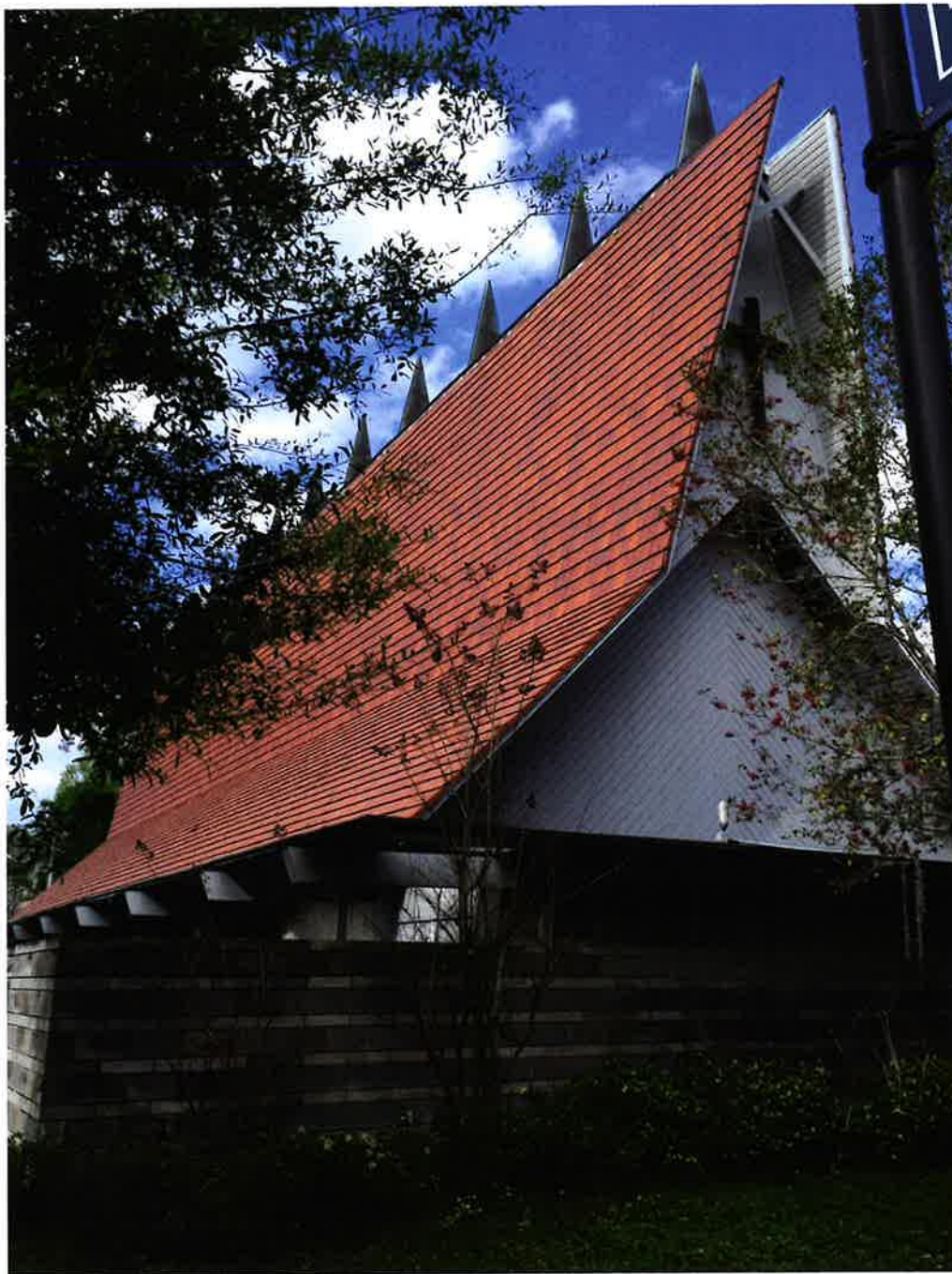
Figure 6. University Evangelical Lutheran Church, Ludovici tile roof. Image Sujin Kim, photographed September 7, 2016.
