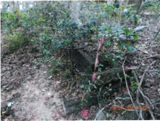
3/1/2018 North Florida Regional Medical Center Photo 5-DSCN2769.JPG
