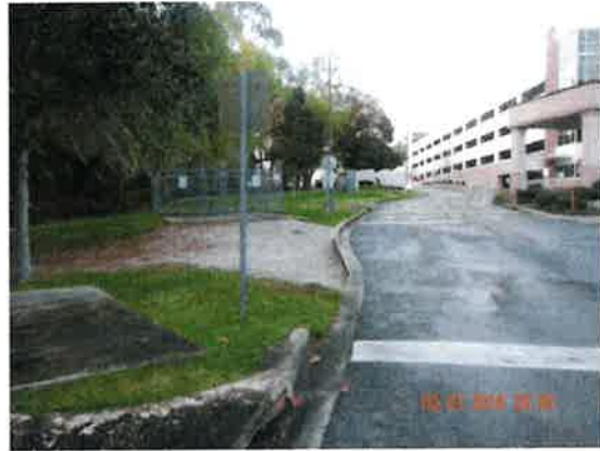
3/1/2018 North Florida Regional Medical Center Photo 34-DSCN2798.JPG
