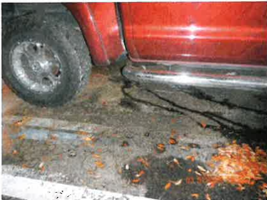
3/1/2018 North Florida Regional Medical Center Photo 75-DSCN2843.JPG
