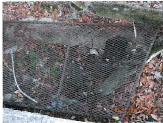
3/1/2018 North Florida Regional Medical Center Photo 16-DSCN2780.JPG
