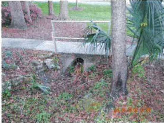
3/1/2018 North Florida Regional Medical Center Photo 13-DSCN2777.JPG
