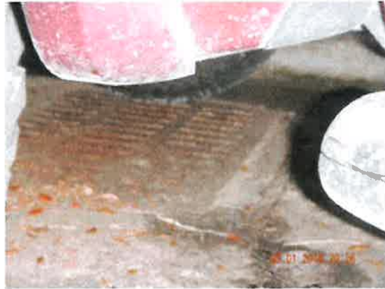
3/1/2018 North Florida Regional Medical Center Photo 76-DSCN2844.JPG
