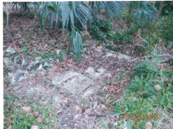
3/1/2018 North Florida Regional Medical Center Photo 12-DSCN2776.JPG
