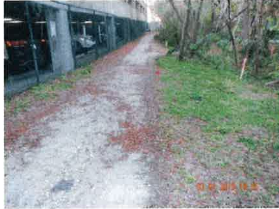
3/1/2018 North Florida Regional Medical Center Photo 14-DSCN2778.JPG
