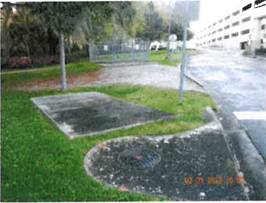
3/1/2018 North Florida Regional Medical Center Photo 29-DSCN2793.JPG
