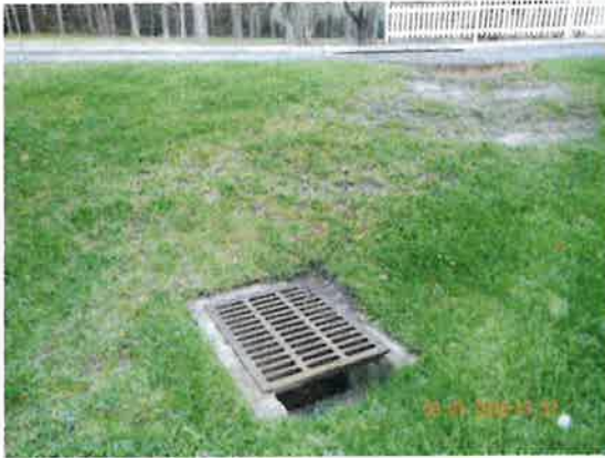
3/1/2018 North Florida Regional Medical Center Photo 21-DSCN2785.JPG
