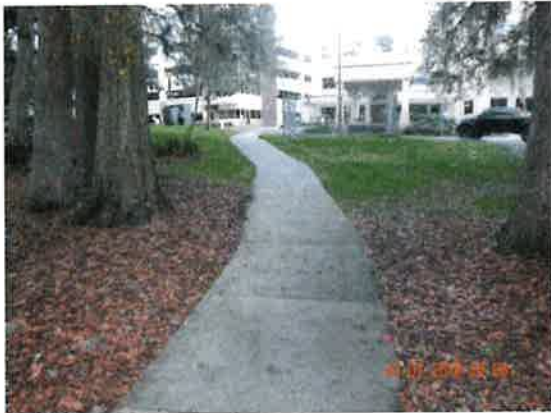
3/1/2018 North Florida Regional Medical Center Photo 39-DSCN2803.JPG
