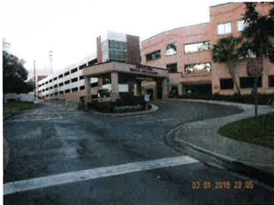
3/1/2018 North Florida Regional Medical Center Photo 35-DSCN2799.JPG
