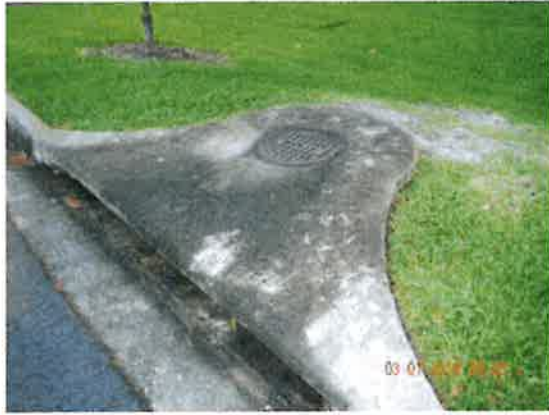
3/1/2018 North Florida Regional Medical Center Photo 32-DSCN2796.JPG
