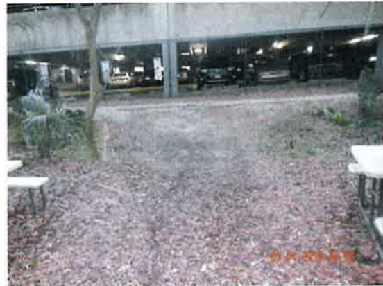
3/1/2018 North Florida Regional Medical Center Photo 36-DSCN2800.JPG
