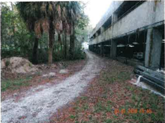
3/1/2018 North Florida Regional Medical Center Photo 1-DSCN2765.JPG
