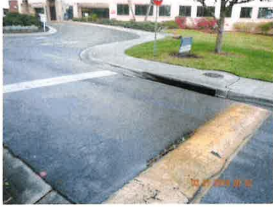
3/1/2018 North Florida Regional Medical Center Photo 30-DSCN2794.JPG
