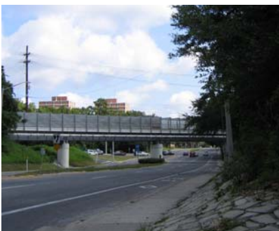
Depot Avenue Rail Trail crossing over 13 th Street
