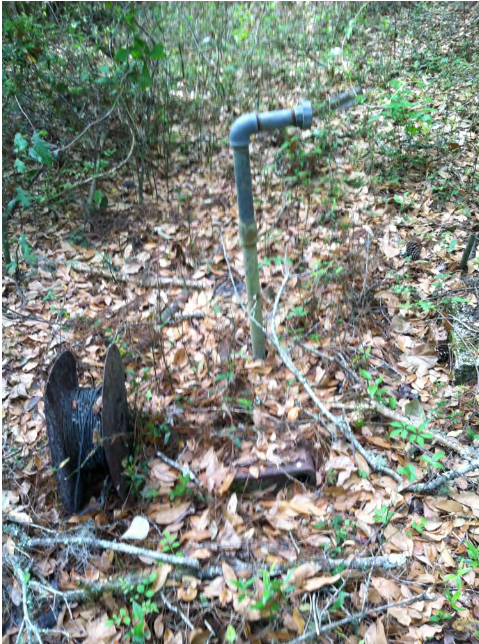
View of suspected water well on subject property
