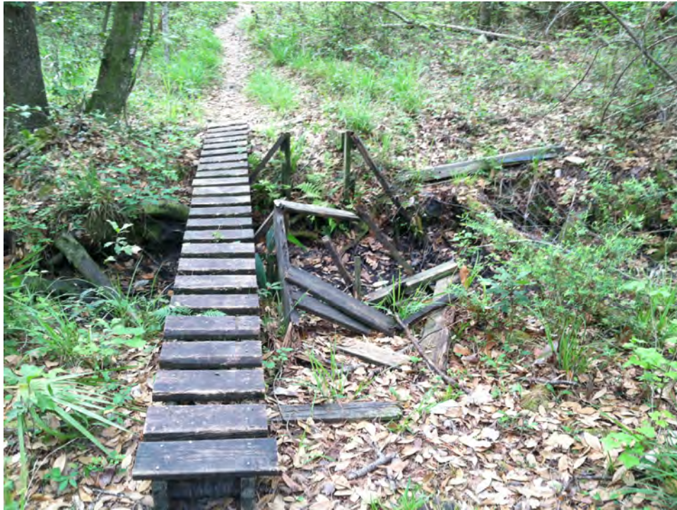
View of foot bridge on subject property
