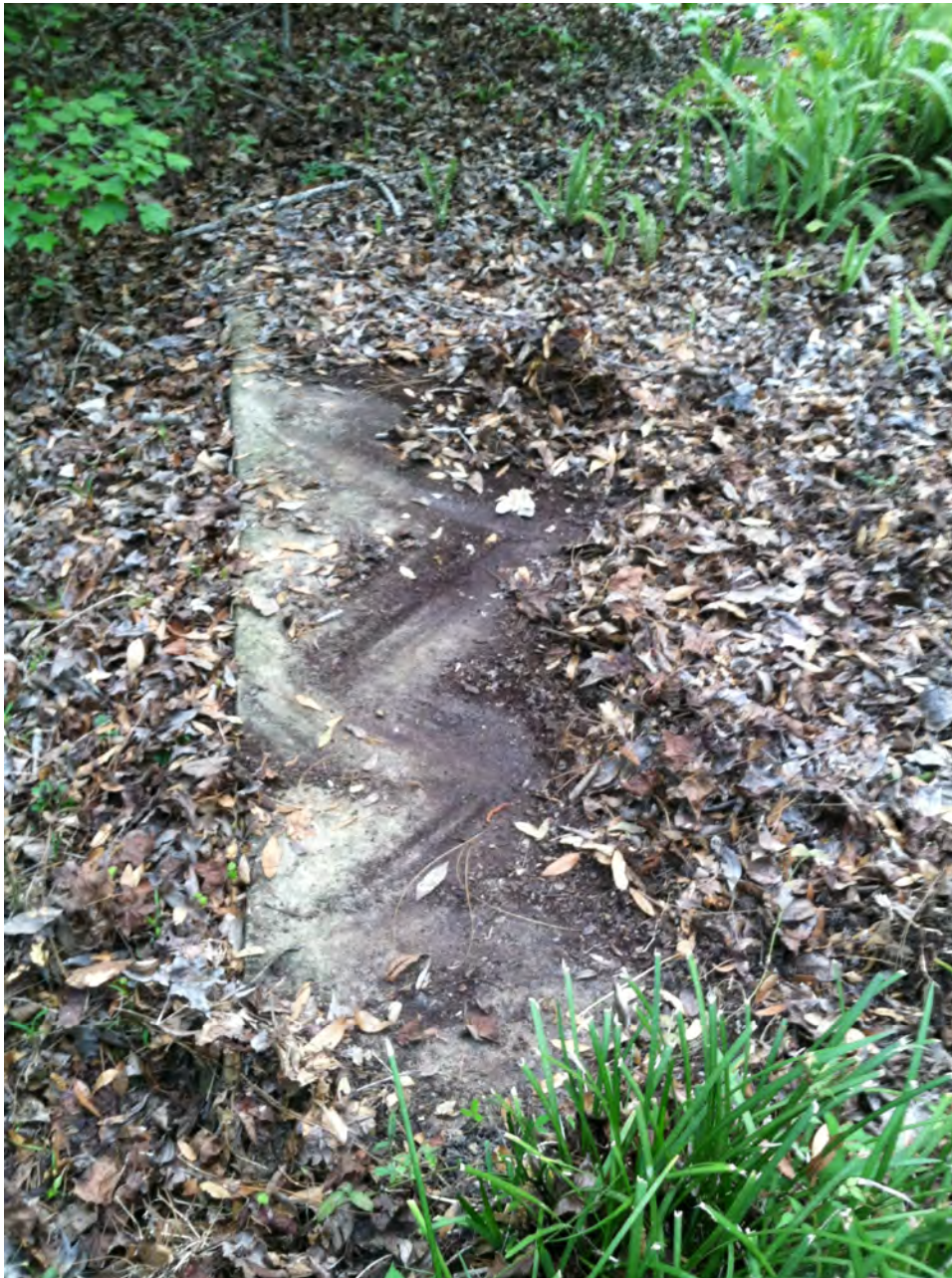
View of one of the concrete pads on subject property
