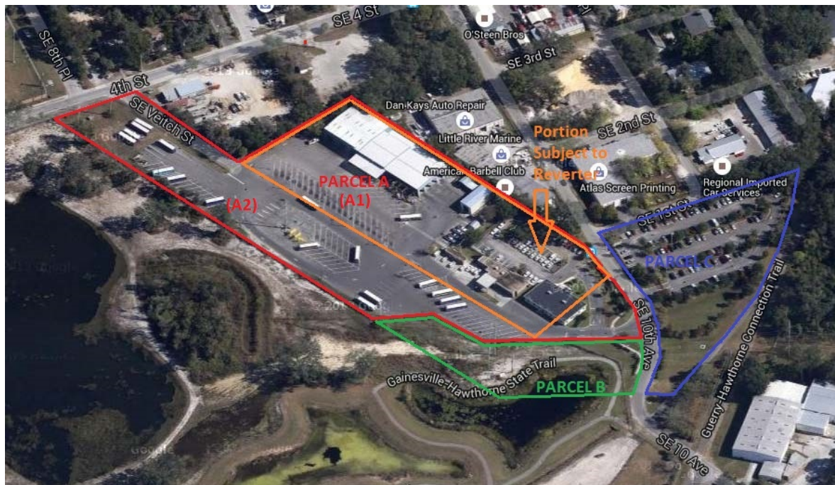
Figure1. - RTS Original Facility
