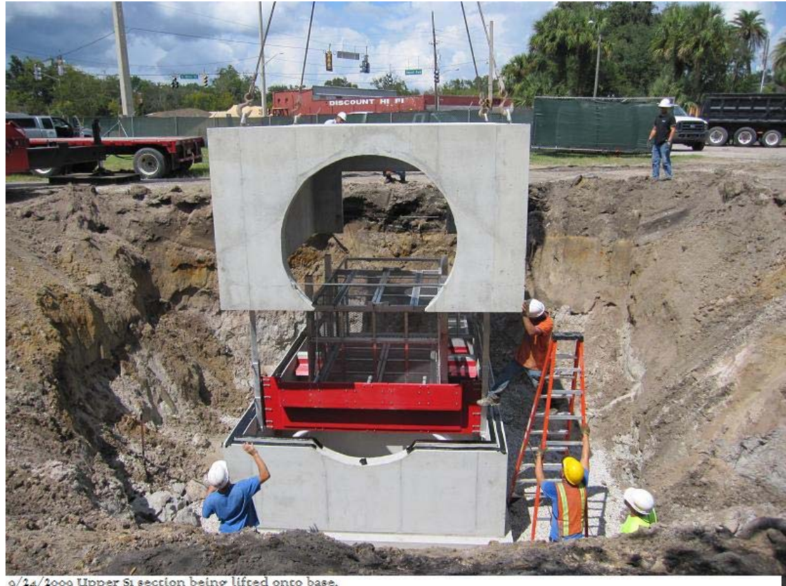
9/14/2000 Upper S1 section being lifted onto base.
