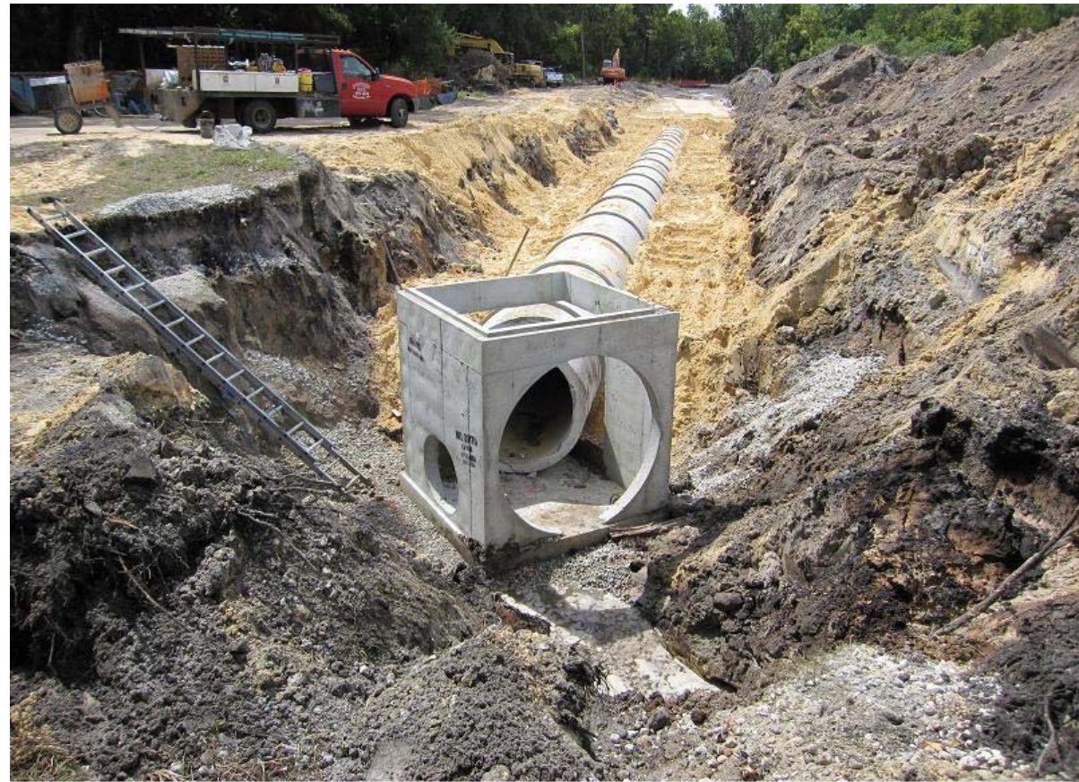
9/17/2009 (pm) S26 J-box installation facing SSW
