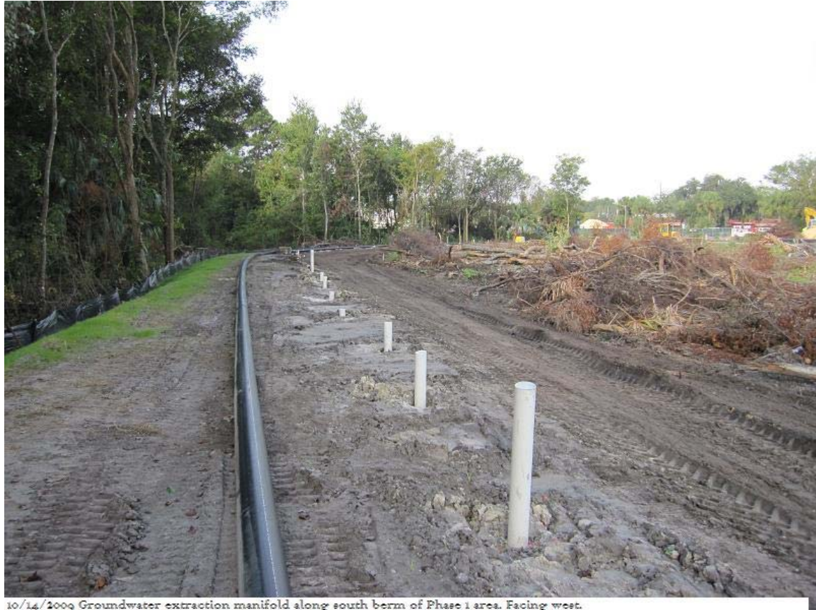
10/14/2009 Groundwater extraction manifold along south berm of Phase 1 area. Facing west.
