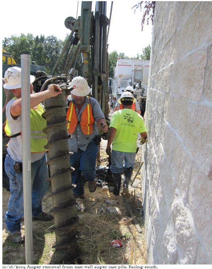
10/16/2009 Auger removal from east wall auger cast pile. Facing south.
