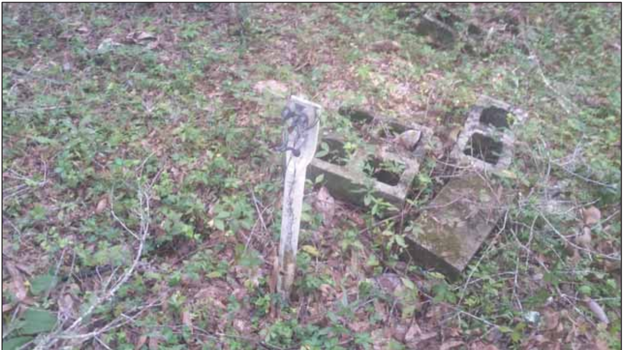
Figure 38. An old electrical junction located in the north central portion of the study site.
