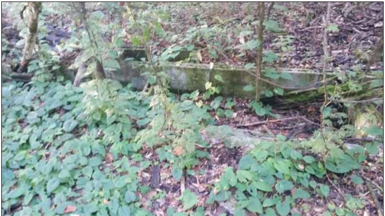
Figure 30. Old foundation located in the parcel 06949-000-000
