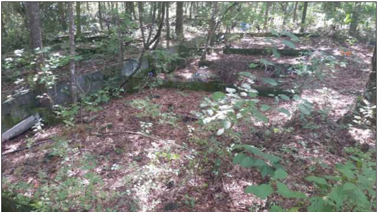
Figure 32. Old foundation located in the central portion of the study site.
