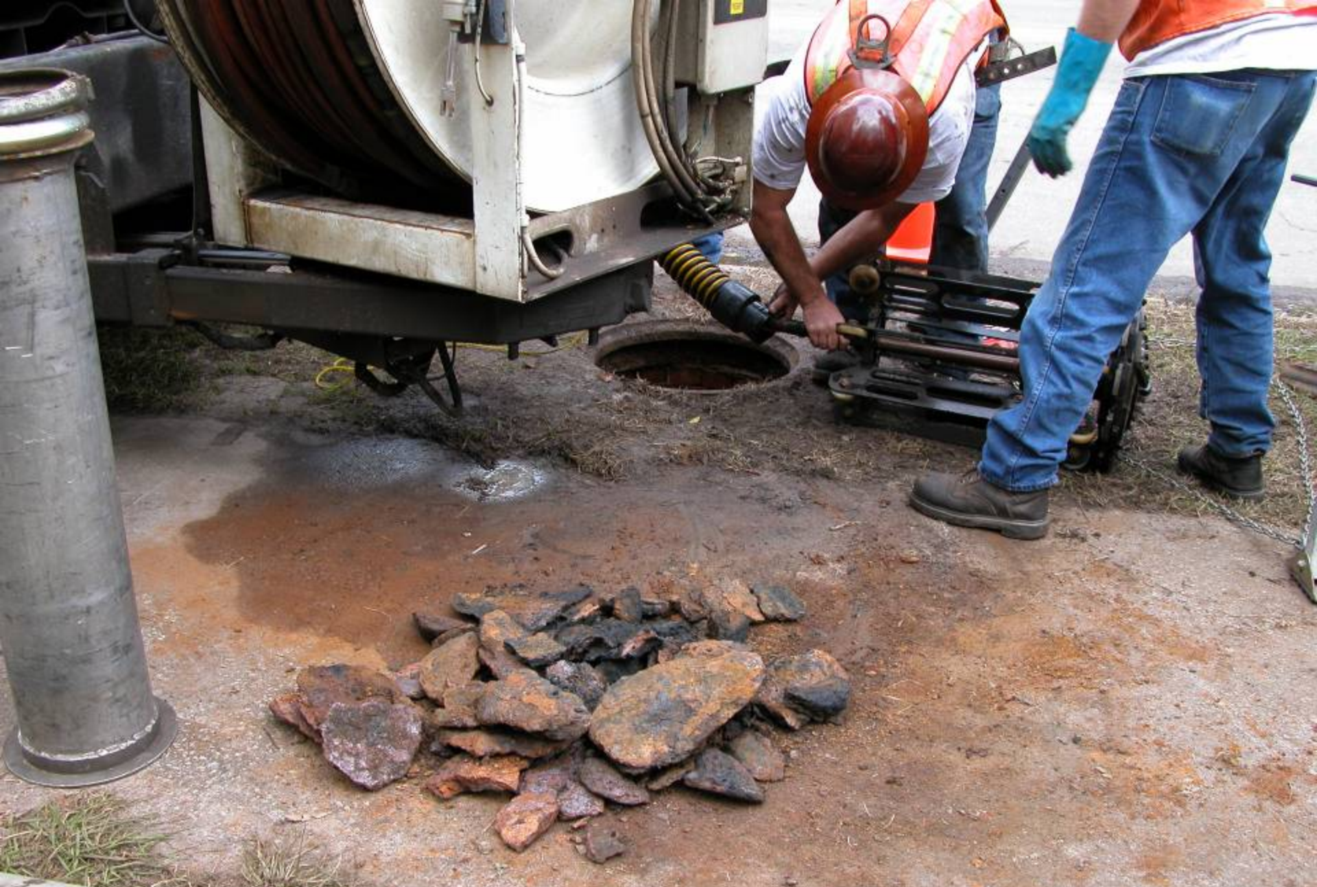
Tuberculation Removed with Hydraulic Chain Cutter
