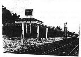
Bergmann Associates recently completed construction documents for Phase 1 of this project, which includes the structural rehabilitation of the existing 80 year-old historic timber-framed train platform canopy, and other improvements such as sidewalks, curbs, planters, canopy roof drainage improvements, and other amenities.
