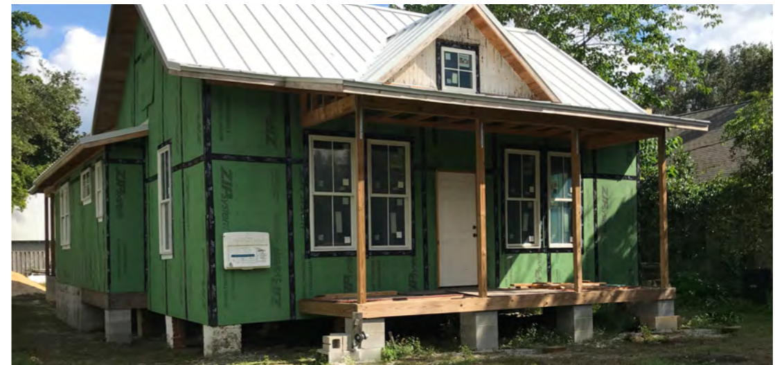
Photo of current stage of renovations:
