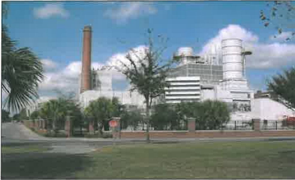
J. R. Kelly Generating Station
