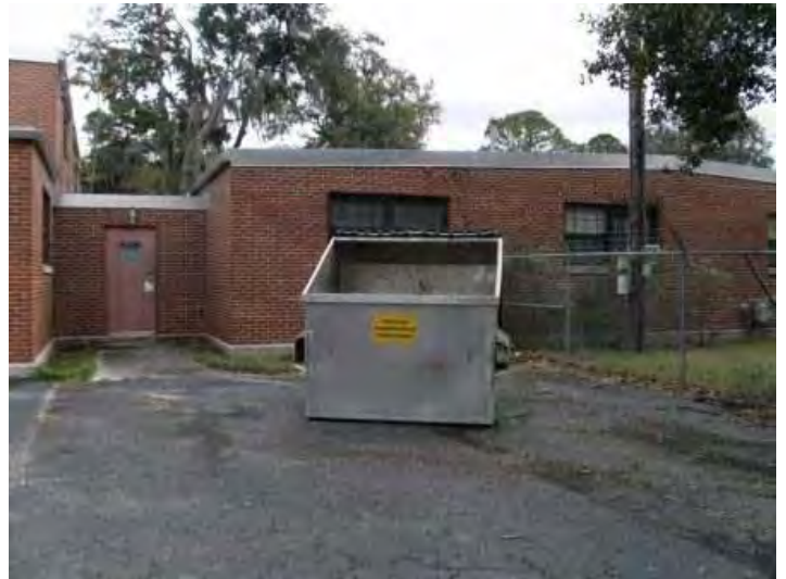
Solid Waste Dumpster
