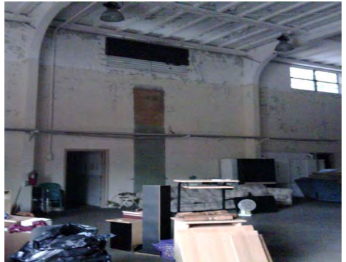
Drill Hall in Administration Building
