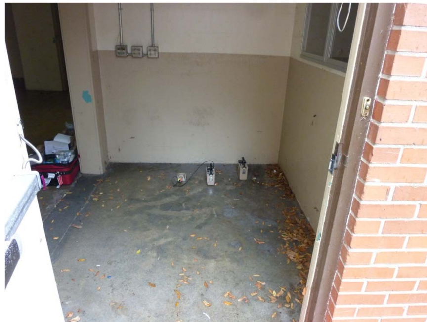
Layton USARC_Background entryway near rollup door
