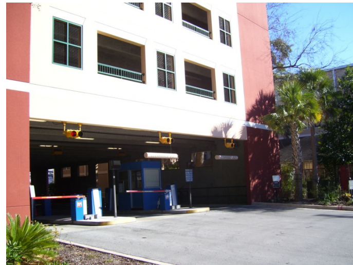
City Parking Garage
