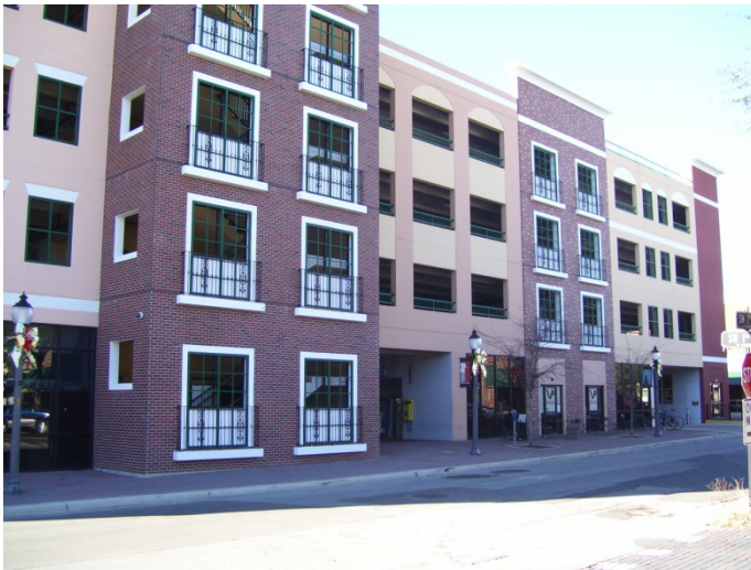
City Parking Garage
