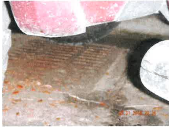
3/1/2018 North Florida Regional Medical Center Photo 76-DSCN2844.JPG
