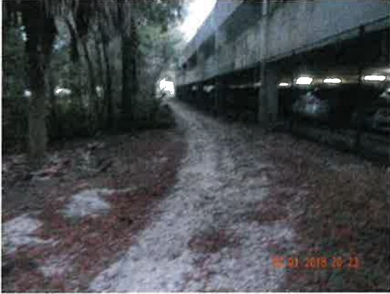
3/1/2018 North Florida Regional Medical Center Photo 69-DSCN2837.JPG
