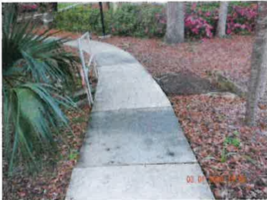
3/1/2018 North Florida Regional Medical Center Photo 15-DSCN2779.JPG
