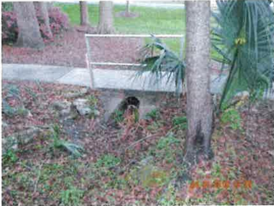
3/1/2018 North Florida Regional Medical Center Photo 13-DSCN2777.JPG
