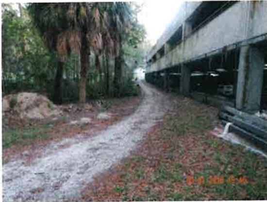
3/1/2018 North Florida Regional Medical Center Photo 1-DSCN2765.JPG
