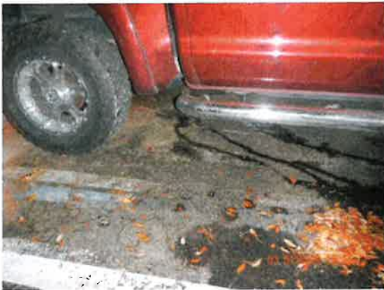
3/1/2018 North Florida Regional Medical Center Photo 75-DSCN2843.JPG
