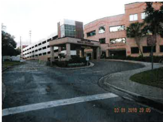
3/1/2018 North Florida Regional Medical Center Photo 35-DSCN2799.JPG
