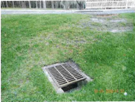
3/1/2018 North Florida Regional Medical Center Photo 21-DSCN2785.JPG
