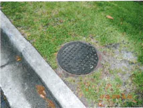
3/1/2018 North Florida Regional Medical Center Photo 31-DSCN2795.JPG
