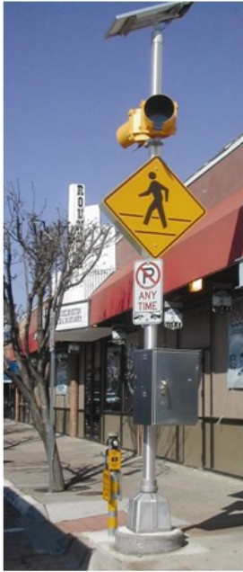
Figure 7: Flashing Beacon
