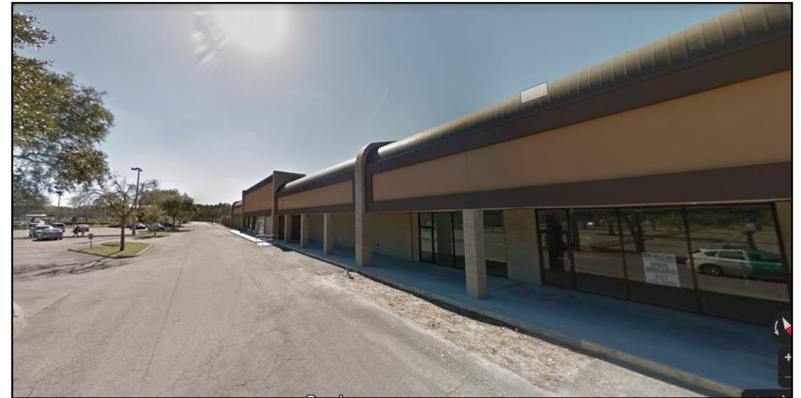
Vacant Northwood Village in Gainesville, with potential for reuse and redevelopment
