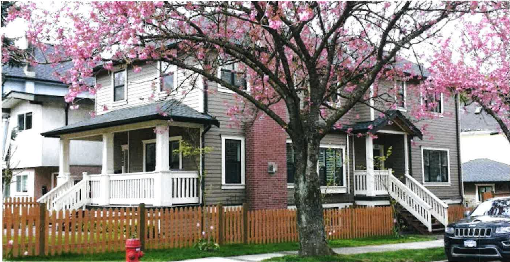
Example of duplex housing. (City of Vancouver)
