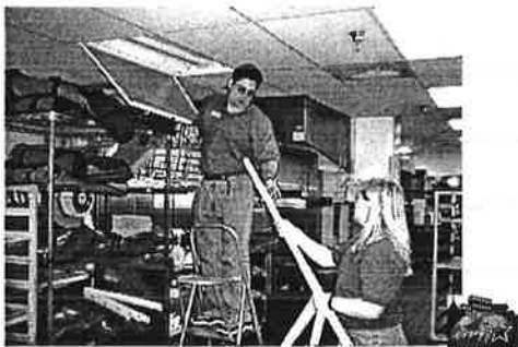
US EPA Green Lights™ 4-lamp T-12 fluorescents can be retrofitted to 2-lamp T-10s, reducing lighting costs by 50%.
