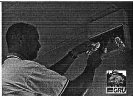
US EPA Green Lights™ Exit signs using light emitting diodes (LEDs) can use 1/20 the energy and last 100x as long as incandescent lamps.
