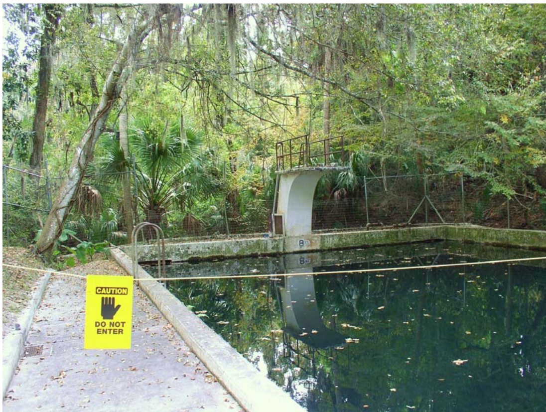
FIGURE 10. VIEW OF GLEN SPRINGS POOL DIVING PLATFORM, FACING SW. (PHOTO BY A. GROSSMAN, 11/22/2010)
