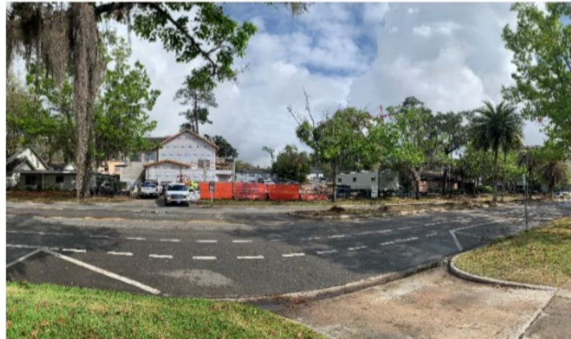
Photo 18. Current construction photo of the restaurant “The Swamp,” a 2-story structure being built to the west of the proposed project, which would be built to the top right of the photo.
