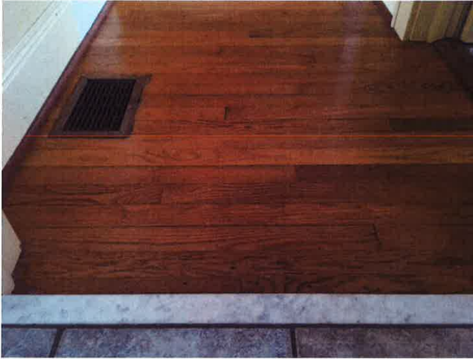
Existing Carrera marble threshold in the hallway
