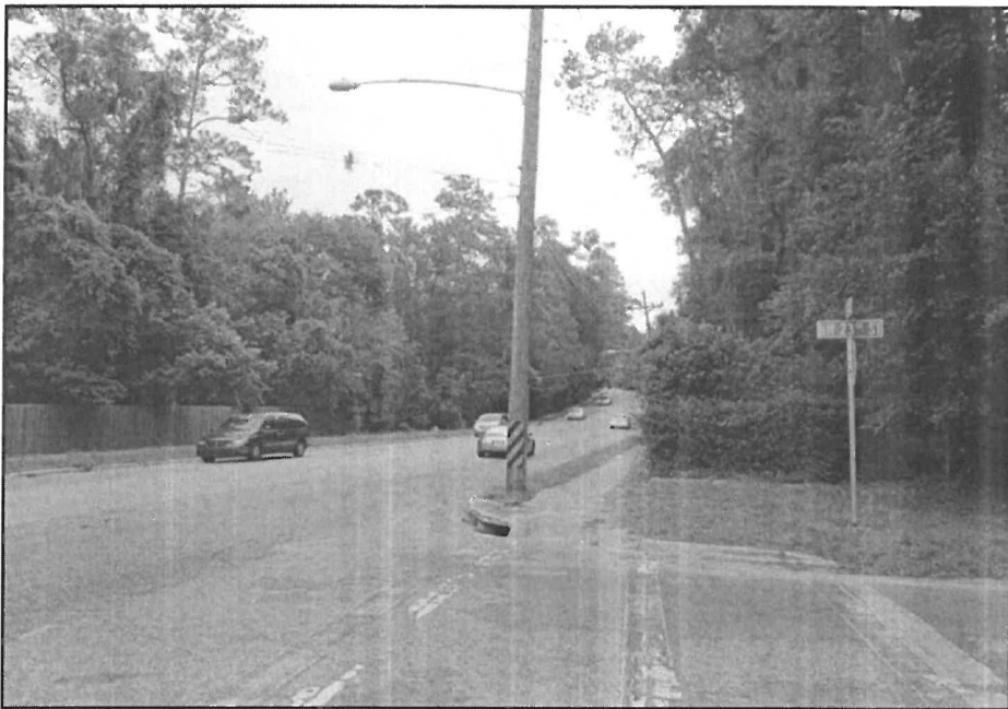
NW 8 th Avenue - view facing east
