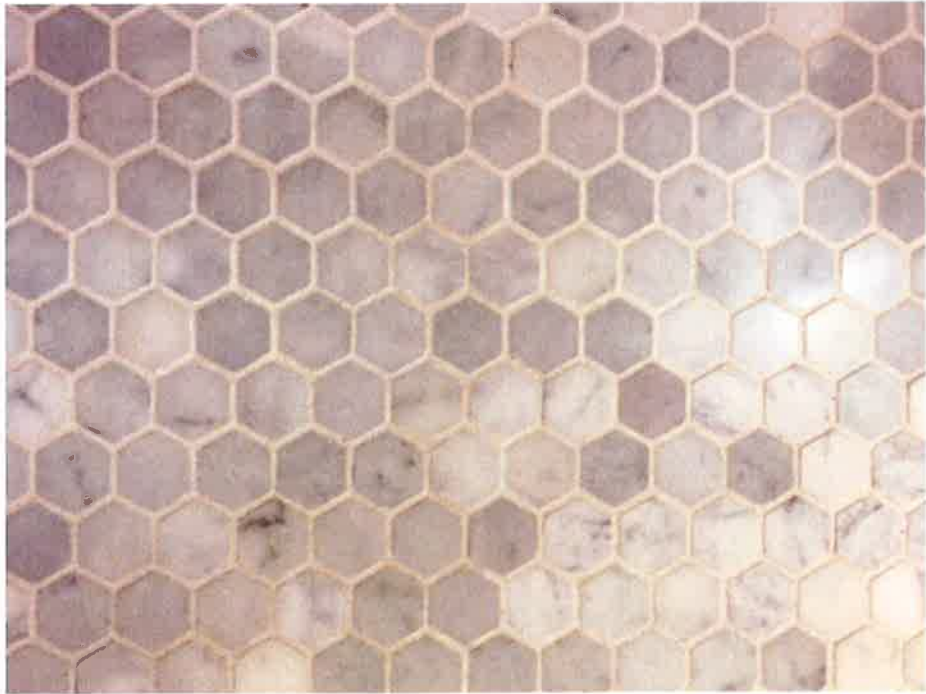
Hexagon Carrera marble subway floor tile in the new bathroom
