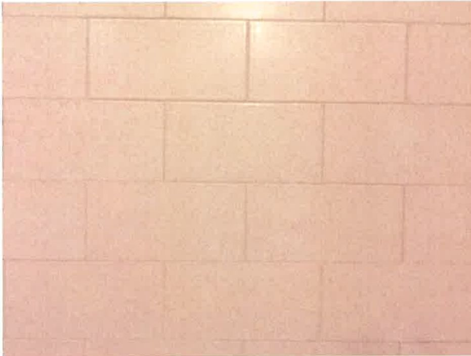
White 3"x6" ceramic subway wall tile in the existing bathroom
