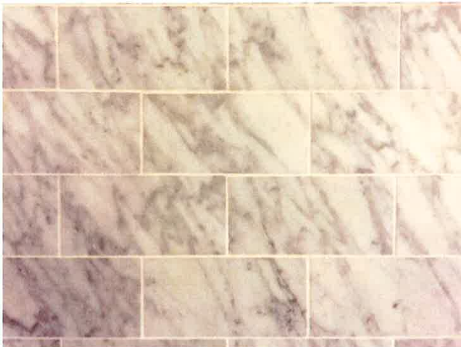
Natural Carrera marble 3"x6" subway wall tile in the new bathroom
