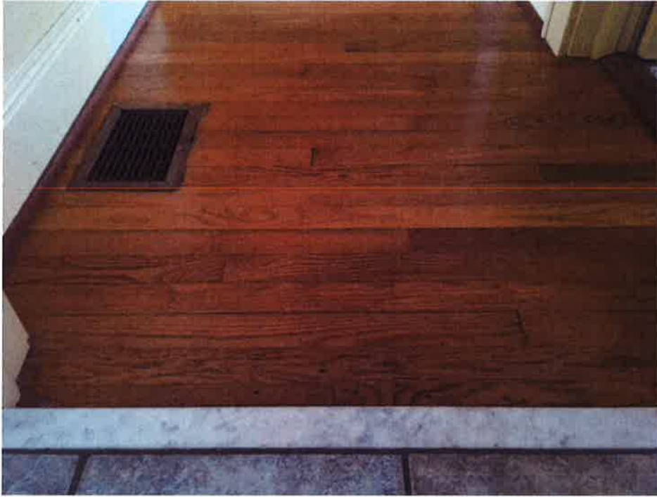
Existing Carrera marble threshold in the hallway
