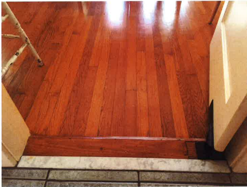
Existing Carrera marble threshold in the dining room
