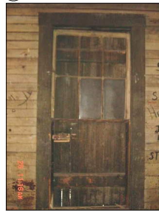
15 INTERIOR PHOTO- WINDOW C A7.2 SCALE: 1 1/2"=1'-0"
