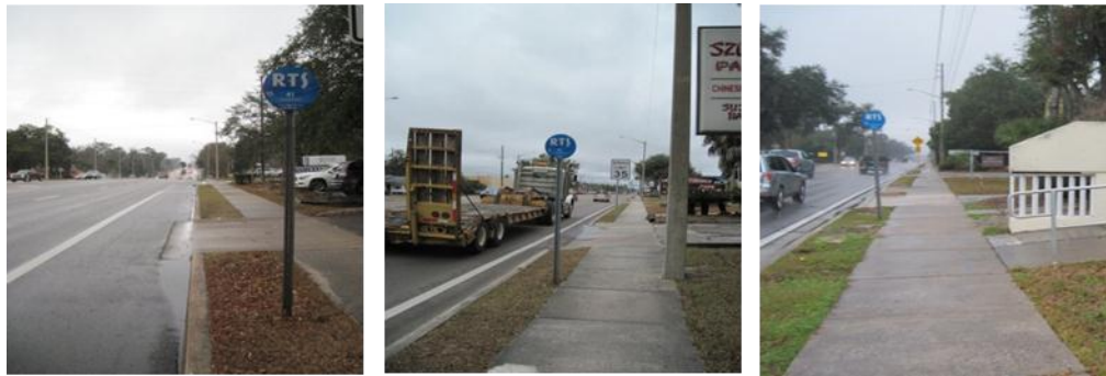
Figure 2-6: Examples of Inadequate Public Transit Facilities
