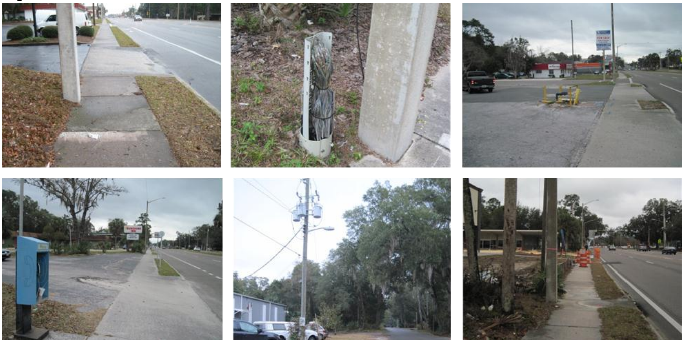
Figure 2-9: Condition of Utilities
