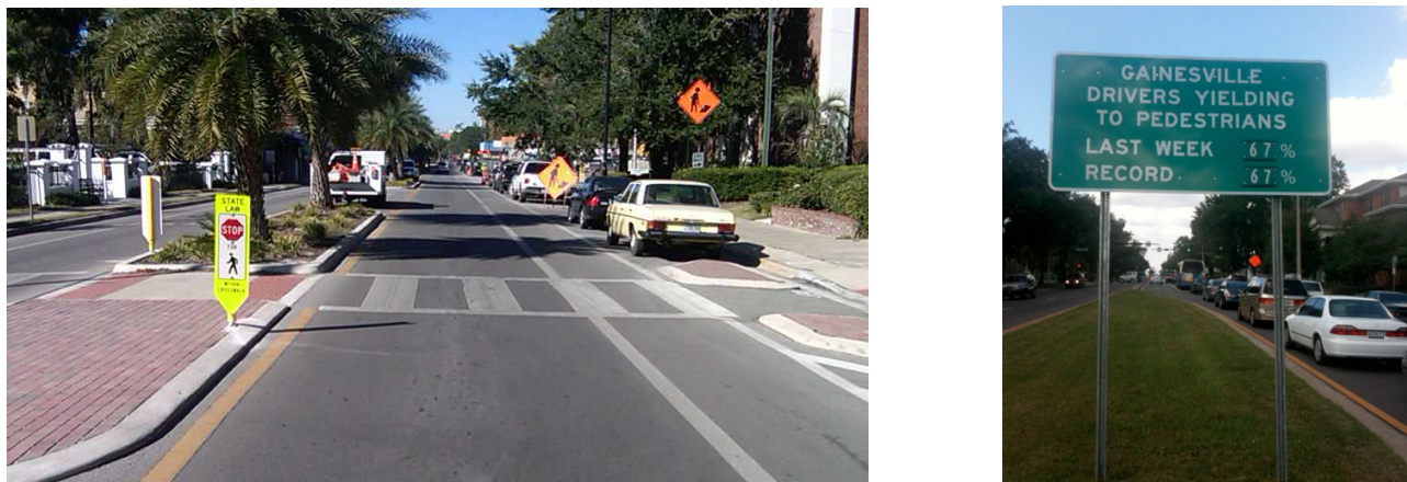
Figure ES-1 Examples of in street crossing and feedback signs
