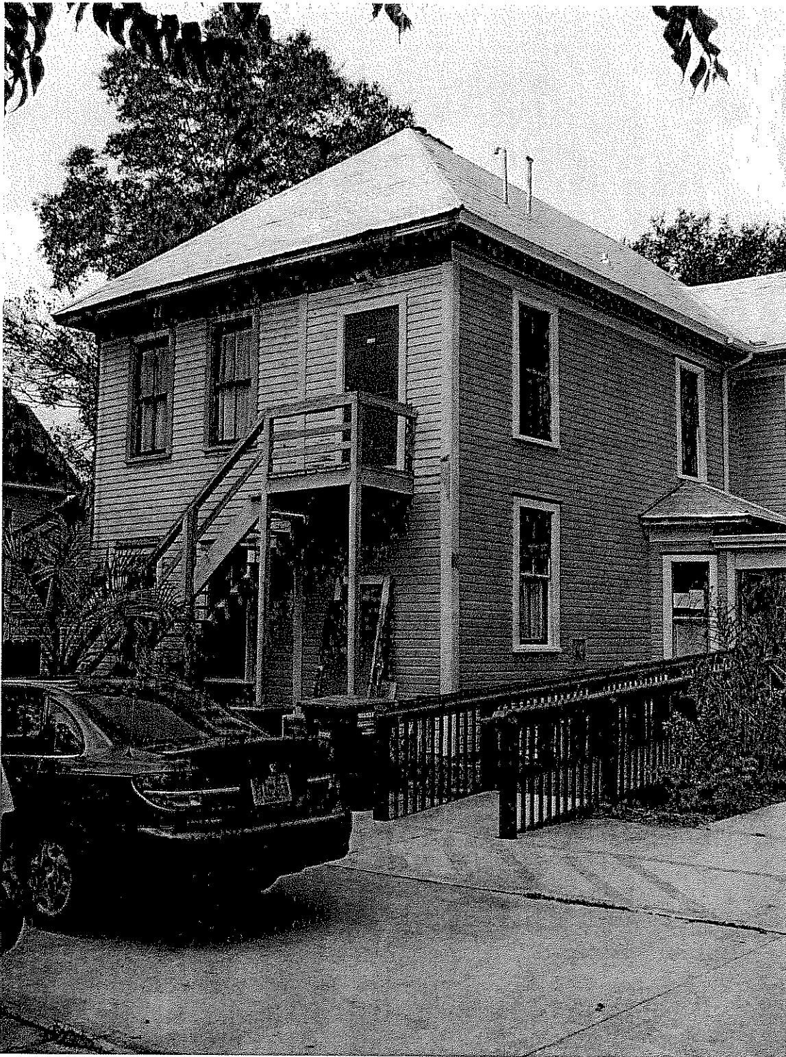
Looking SW from the existing parking lot.
