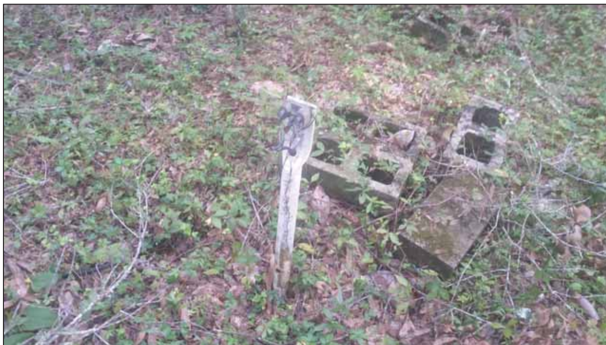
Figure 38. An old electrical junction located in the north central portion of the study site.
