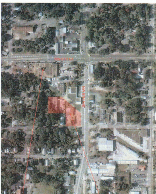
AERIAL SITE VIEW
