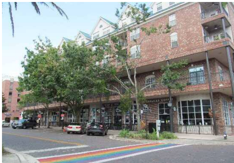
Union Street Station Project – SE 1 st Street
