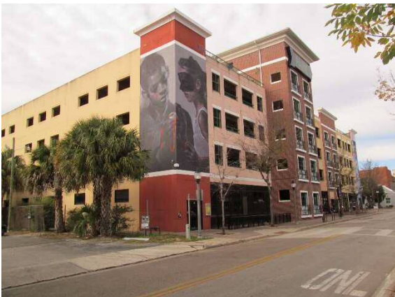
SW Parking garage to the NW
