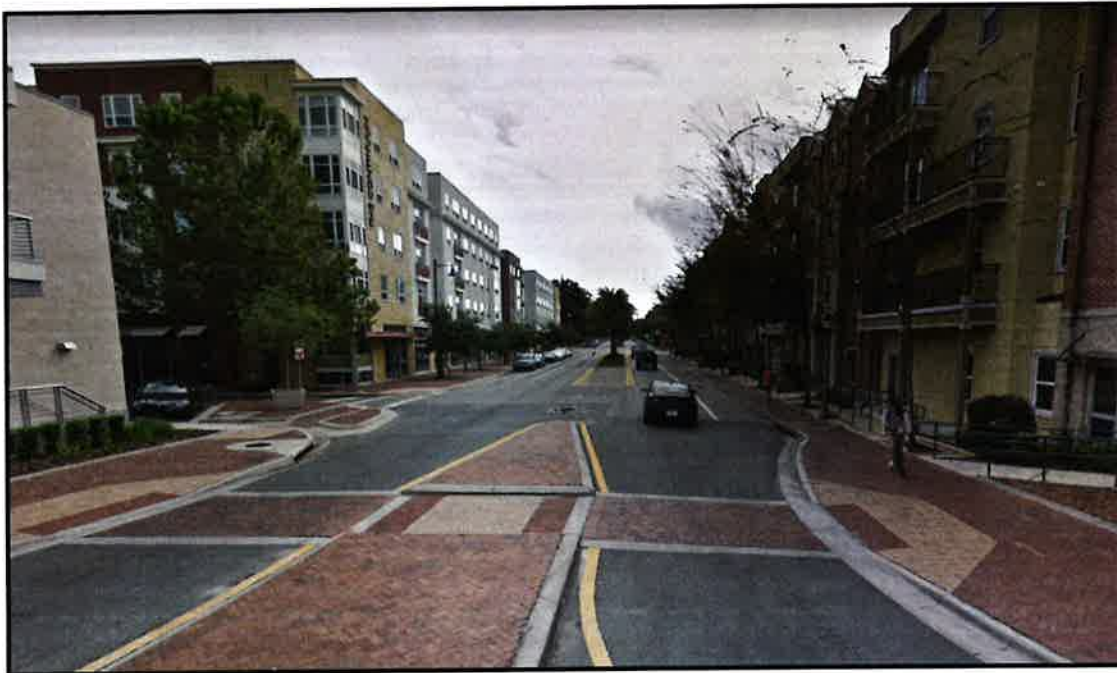
Figure 6: Storefront Street - SW 2 nd Avenue, east of SW 6 th Street
