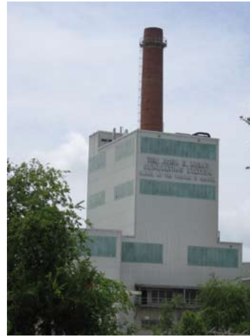
Existing Power Plant
