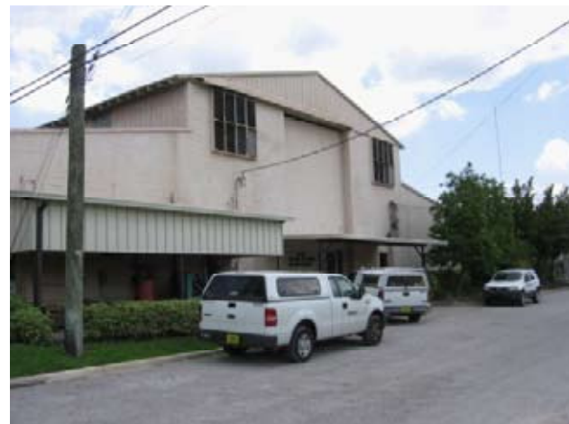
3 Existing GRU Maintenance Building
