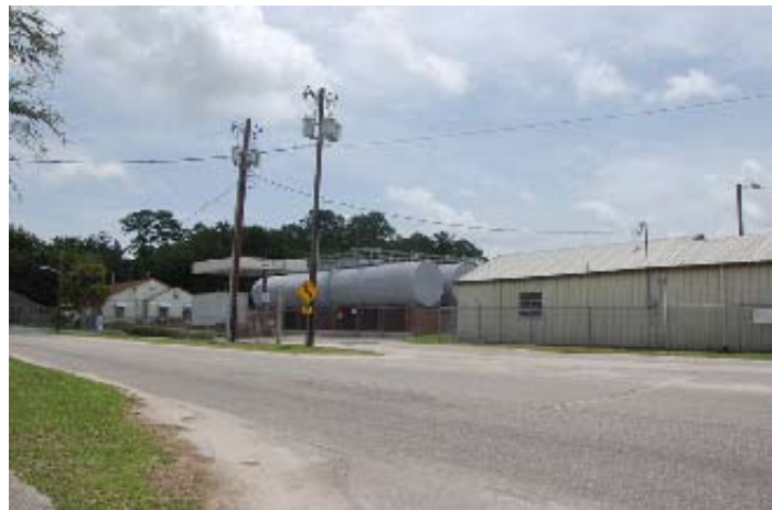
3 Existing Chevron Facility
