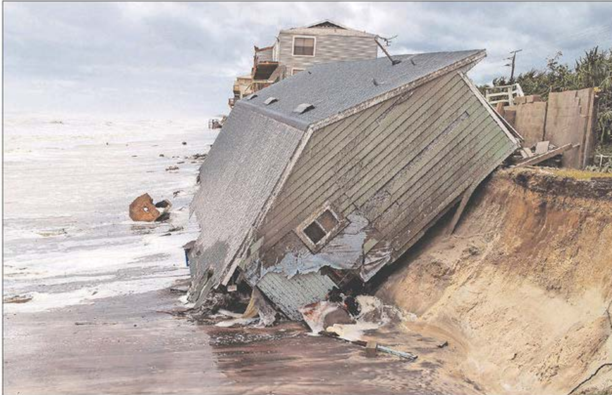
A house slides into the Atlantic Ocean in the aftermath of Hurricane Irma in Ponte Vedra Beach, Monday. [GARY LLOYD MCCULLOUGH/THE FLORIDA TIMES-UNION VIA AP]
