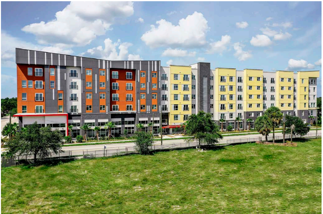
The Salvador Condominiums - 200,000 - SF / St. Petersburg, FL - MEP Design by VoltAir
