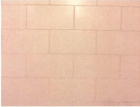
White 3"x6" ceramic subway wall tile in the existing bathroom
