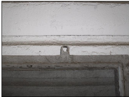
DETAIL PHOTO OF HANGER ASSEMBLY AT HISTORIC REMOVABLE SCREEN INSERT.
