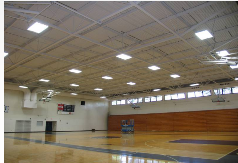
After Energy Efficient Lighting
