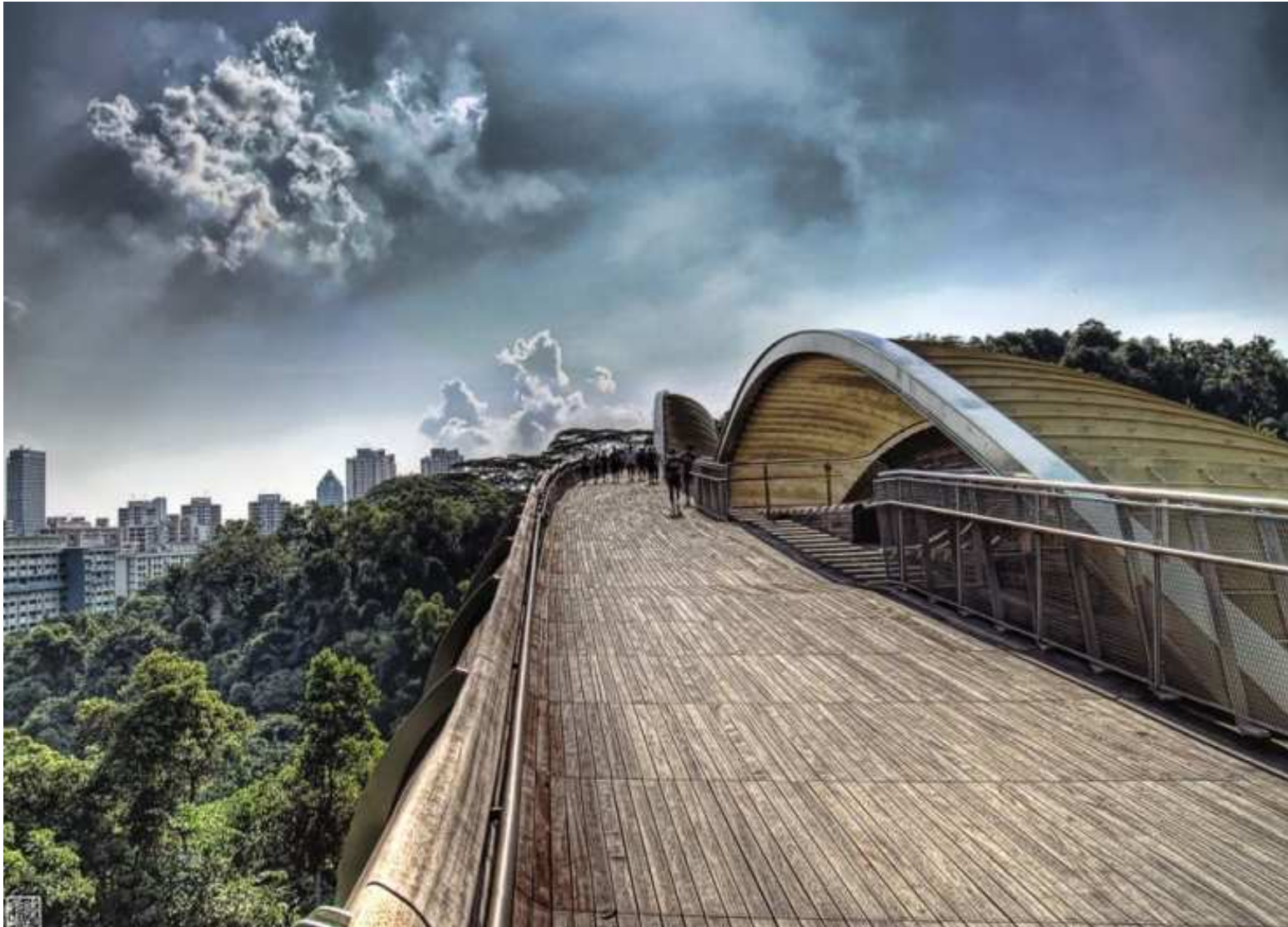
Henderson Waves Pedestrian Bridge, Southern Ridges, Singapore
