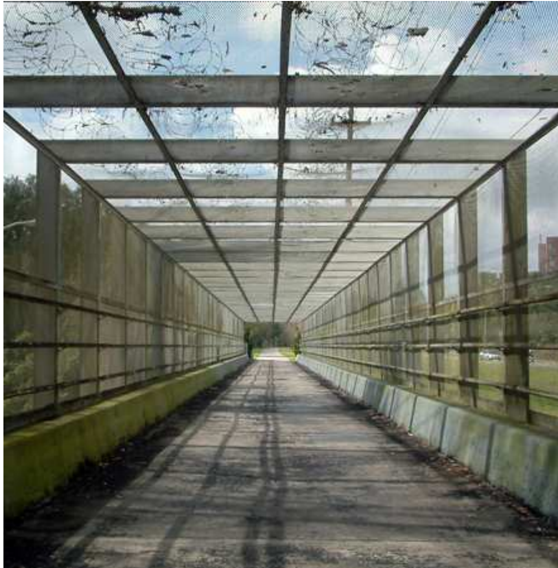
SW 13 th Street Overpass - User experience
