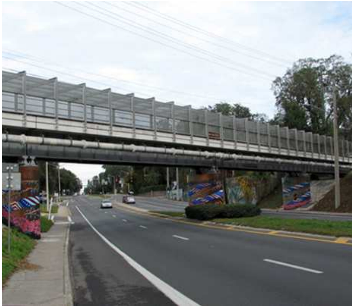
SW 13 th Street Overpass – Gateway into College Park / University Heights
