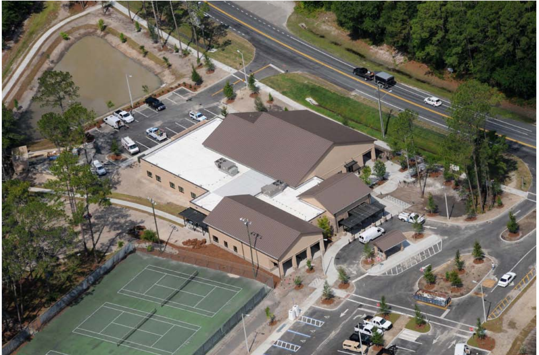
Aerial view looking NNW/Photo taken 6/20/11
