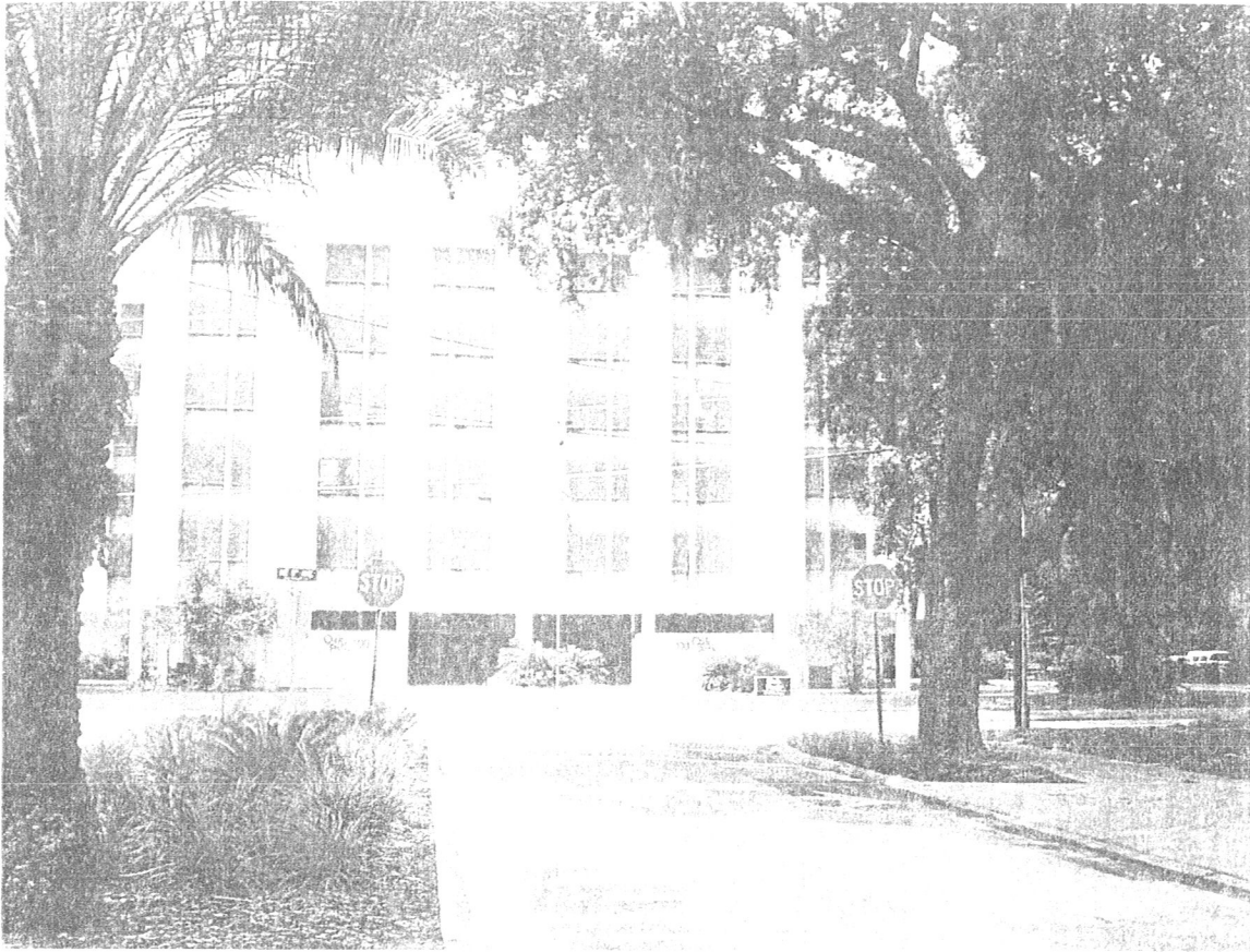
The existing Multi family complex across the street and to the north located on NE 8 th Avenue.
