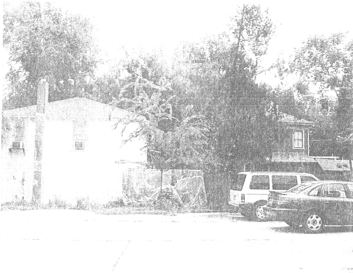
The existing multi-family structure to the rear of the existing parking lot looking east.
