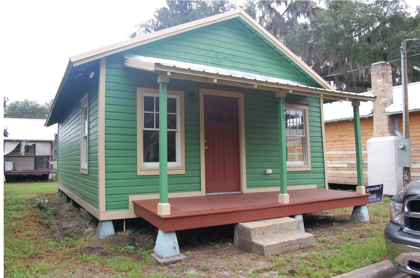
Front (west) facade
