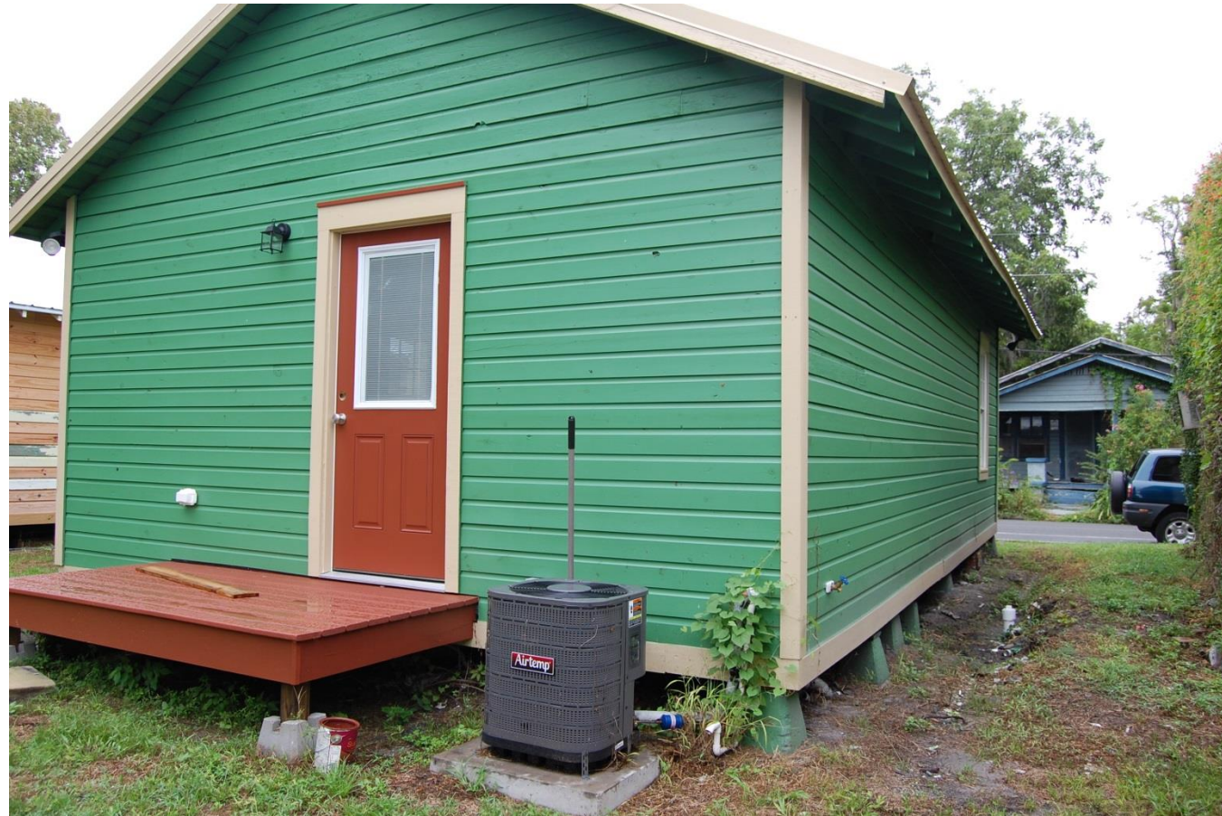
Rear (east) and side (north) facades
